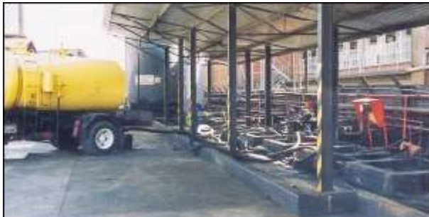
FFS management is committed to environmental improvements at its plants. A new roof over the loading bay at the Teakwood refinery in Durban ducts rain away from the contaminated area to reduce the amount of effluent water to be processed in the plant.
