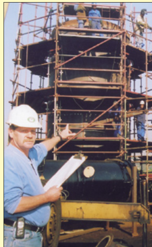
▲ Pressure vessel process tanks under fabrication manager Phillip Vermaak is in the foreground.
