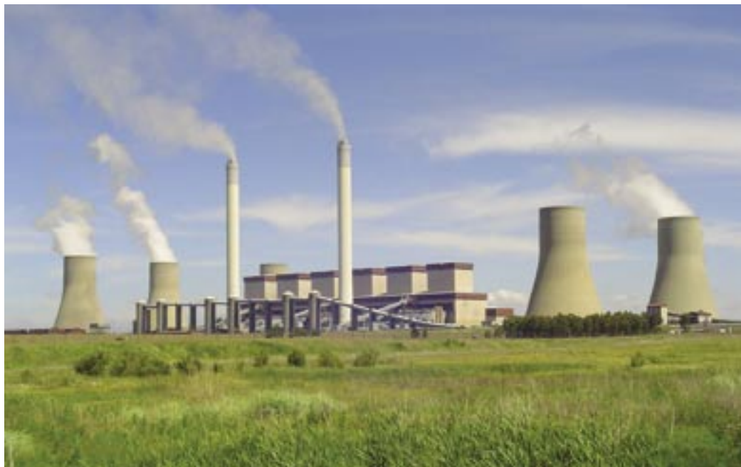
Tutuka Power Station, one of the nine Eskom stations being supplied with FFS industrial heating fuel for start-up purposes.
